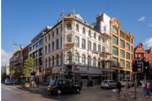
View K: Existing View
