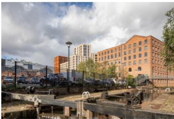
View P: Existing
